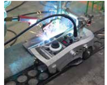
IK-12 NEXT straight welding
