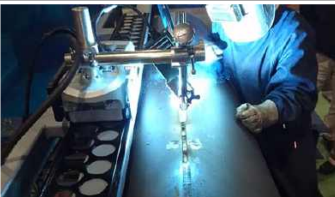
Pipe seam welding with traveling on rail
