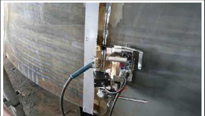
Up-ward pipe welding
